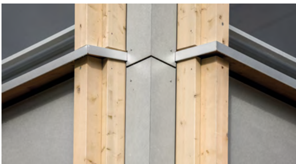
Visible mounting combined with the Closed Corner 90° system
