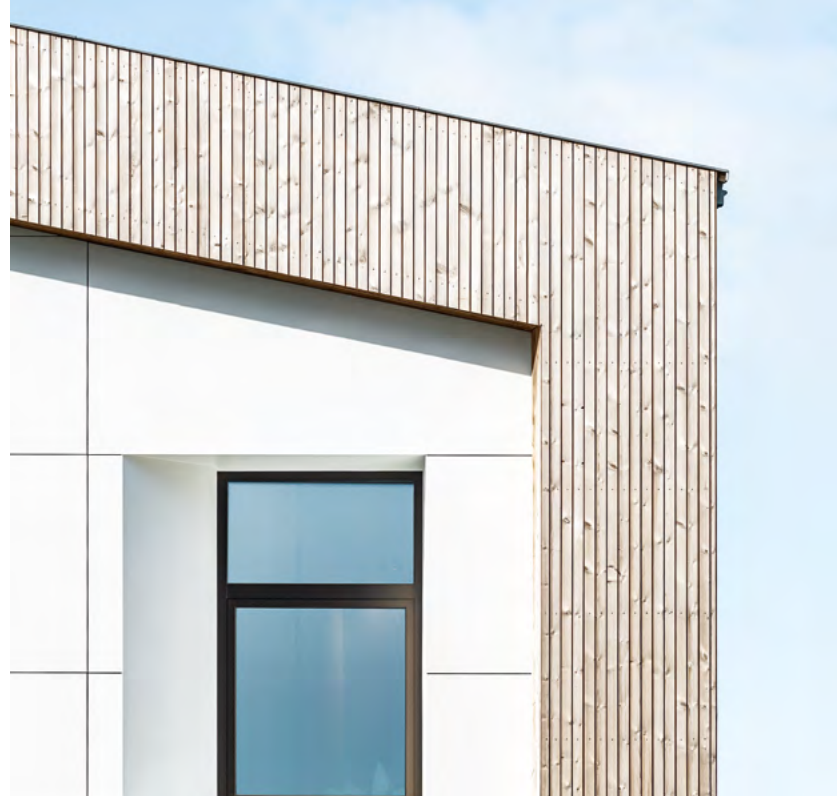
Invisible mounting with the Swisspearl Sigma 8 Pro system
