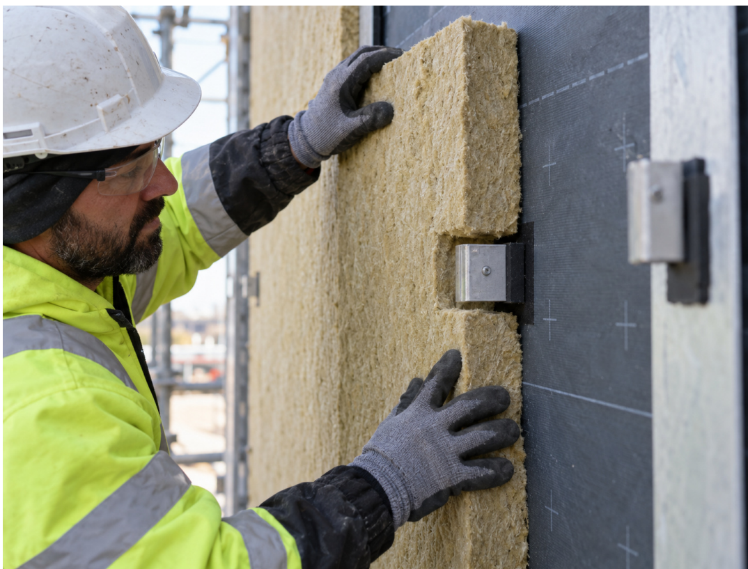
Figure 3 - Mineral Wool Installation Around Subframing
